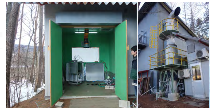
risk assessment experimental facility in Tokyo University of Science at Suwa
