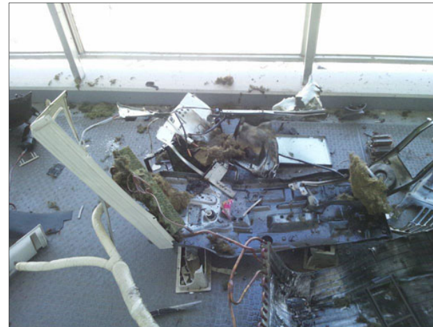
Explosion accident (Tokyo metropolitan government)
