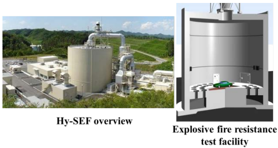
Fig. 5.1 Overview of the Hy-SEF test facility
